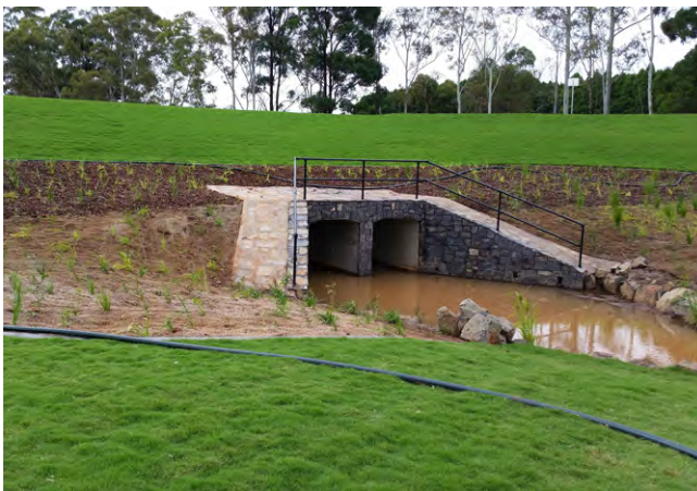
Figure 32: Primary drainage pipes
