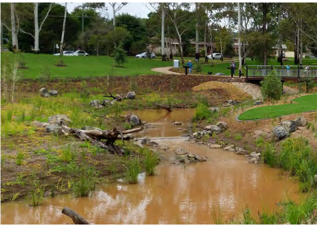
Figure 14: Example natural waterway in a detention basin
