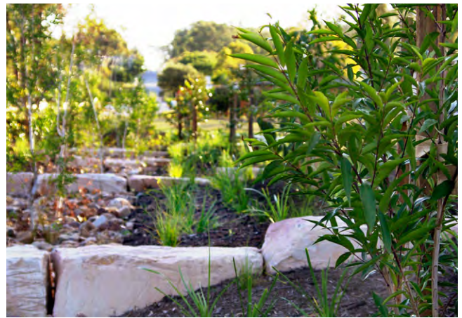
Figure 15: Example dry waterway with small weirs
