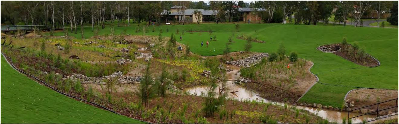
Figure 30: View of detention basin from the top of the earth mound
