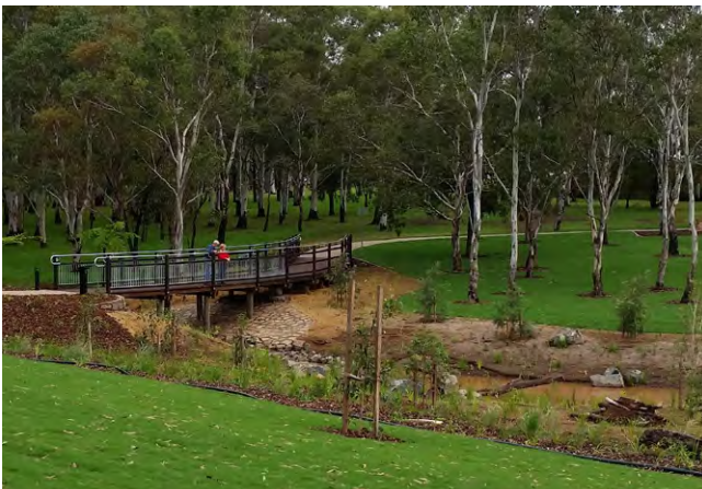
Figure 27: Pedestrian footbridge over waterway
