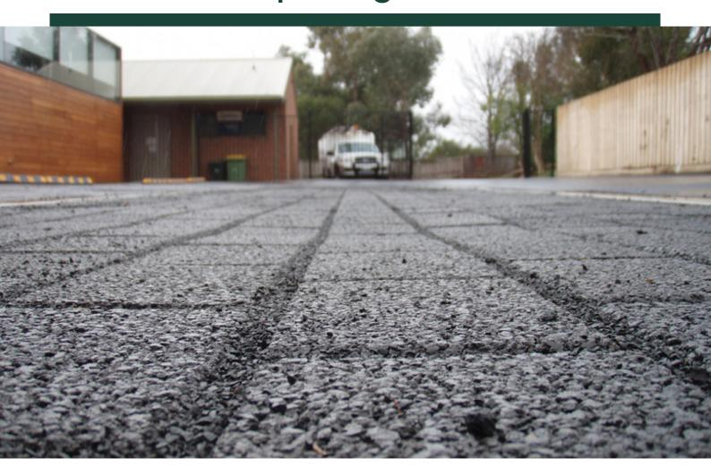
Permeable paving allows water to infiltrate through the paving, reducing the volume of runoff from hard surfaces such as roads, car parks and footpaths. This reduces local flooding and surface ponding, and promotes infiltration.
