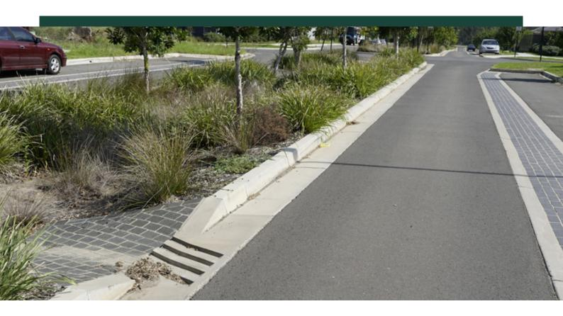
Vegetated buffer strips and swales are simple stormwater transfer systems that treat runoff through filtration and sediment capture. Buffer strips are vegetated surfaces (usually grassed) that allow runoff to flow towards a downstream outlet. Swales generally form a sloped vegetated channel that conveys stormwater along a long path. In both systems, water is slowed and filtered as it flows through the vegetation, capturing large sediments and absorbing stormwater runoff.
