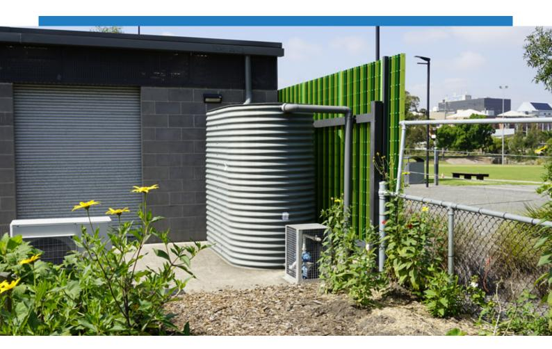
A rainwater tank captures and stores roof water for reuse on-site. It may also play a part in local flood control.
