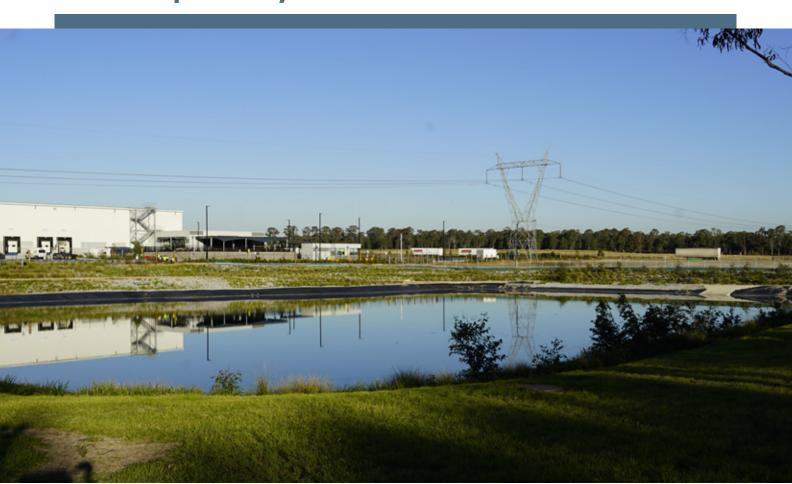
Temporary sediment basins are installed during the construction stage of a development to help manage stormwater impacts during construction. These open water bodies treat stormwater by allowing coarse particles and suspended sediments to settle.
