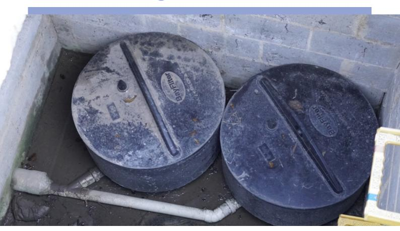
Filter cartridges include sand filters and proprietary products that operate in a similar way to GPTs, but are designed to filter finer pollutants, such as fine solids, soluble heavy metals, oils and nutrients.
