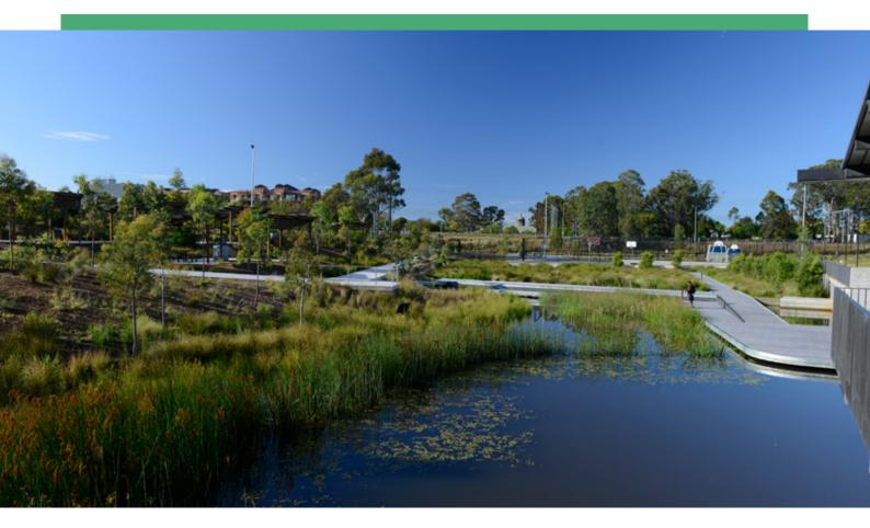
A wetland is a vegetated wet basin (or series of wet basins) that filter and treat stormwater before it enters our waterways. The plants in a wetland capture fine particles and absorb nutrients from the stormwater; they slow and filter the water allowing sediment to settle. Wetlands commonly have a gross pollutant and sediment trap upstream of them to capture coarse material before it enters the main part of the wetland (the macrophyte zone).
