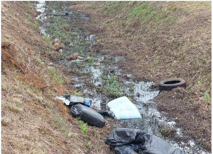
Image 2. Waste dumped in a drainage channel.
