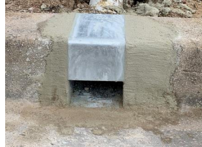
Figure 17 Galvanised full kerb height steel private stormwater outlet adaptor
