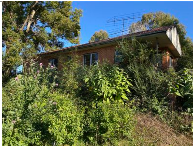
Photograph 15: Rear of house. View to west.
