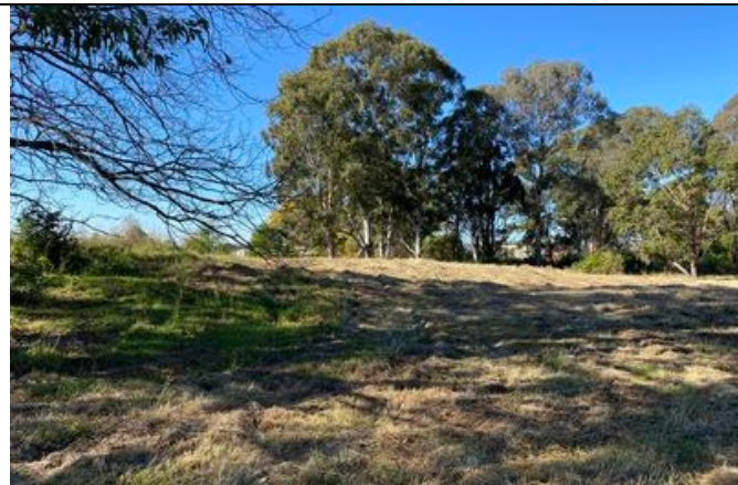
Photograph 10: Raised levee on southern side of canal. View to NE
