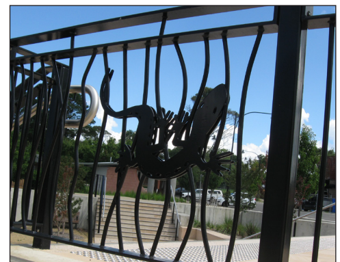
Lawson Town Centre - custom railing
