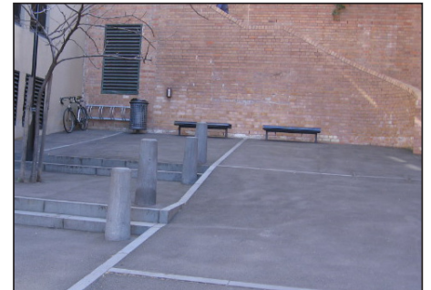
Change of level well integrated into public domain - precast steps, The Rocks
