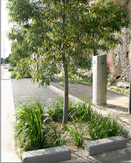
Tree planting in carriageway with raingarden
