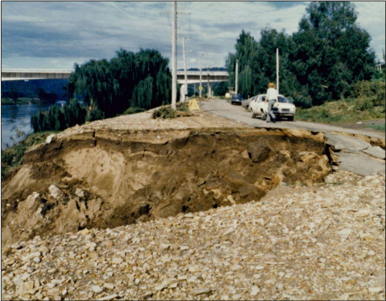
Plate 4: Willows and erosion adjacent River Road in 1978 (Photo courtesy: Penrith City Council)
